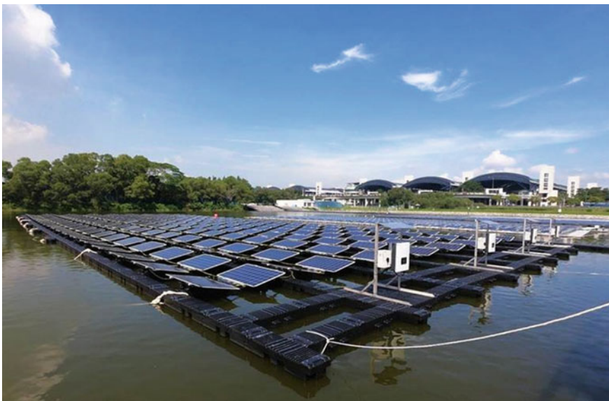
Fig. 16 Constructed floating solar farm at Tengeh reservoir
