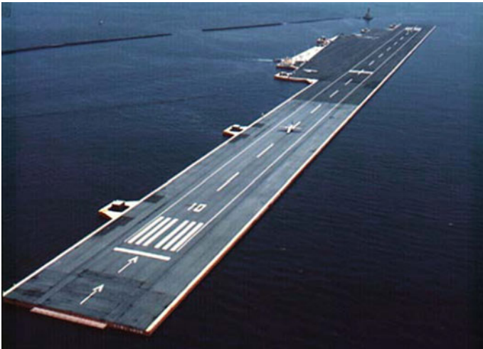
Fig. 28 Mega-float—a 1 km long floating airplane runway test model in Tokyo Bay. Photo courtesy of M. Fujikubo
