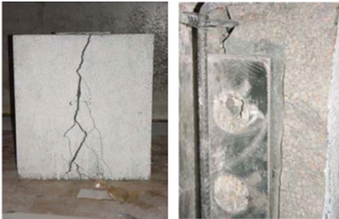
Fig. 14 Cracked slab and deformed perfobond rib at failure
