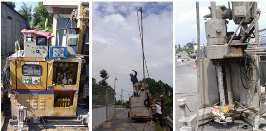
Fig. 2 The secondhand Jet Grouting system used for this study
