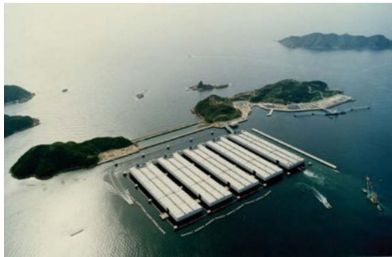
Fig. 6 Kamigoto floating oil storage base
