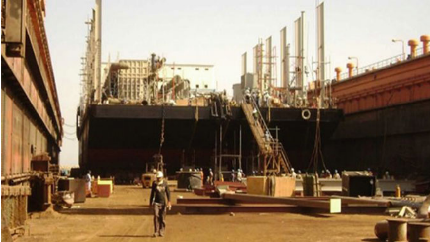
Fig. 8 Floating desalination plant at Jeddah
