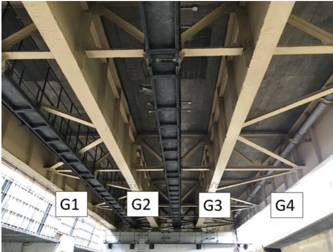
Fig. 5 The test bridge of this study
