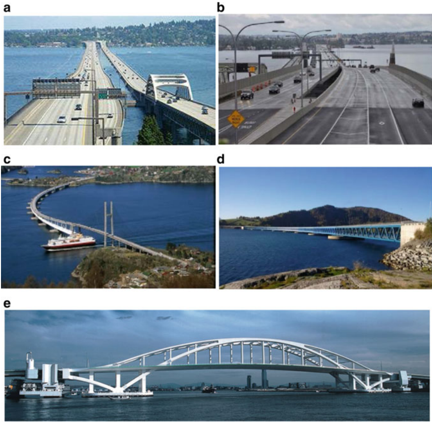
Fig. 26 a Lacey V. Murrow Bridge. b Evergreen point floating bridge. c Nordhordland bridge. d Bergsoysund Bridge. e Yumemai floating steel arch bridge in Osaka
