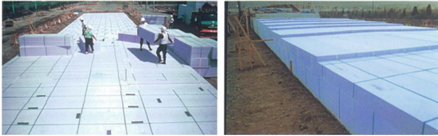
Fig. 1 Road construction using EPS in Japan [3]
