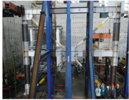
(b) Phase 1 test (1.6% second floor drift)
